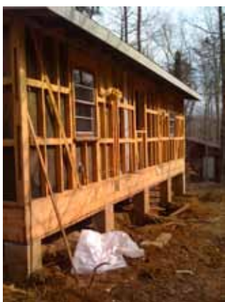
Cabin renovation underway at Lake Cumberland 4-H Camp.
