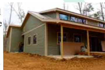
First Cabin of Tomorrow under construction at West KY 4-H Camp.
