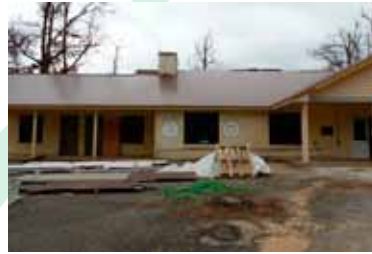
Renovations underway at West KY 4-H Camp to Sparks Hall.
