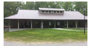
New cabin and storm shelter complex at Feltner 4-H camp.
