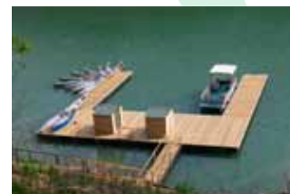
The new dock at the Lake Cumberland 4-H camp.
